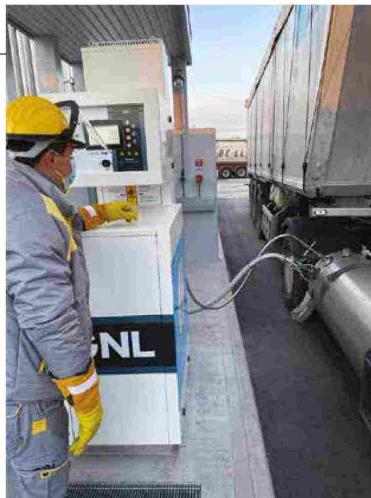
GNL Refuel - Socogas plant, Fidenza
